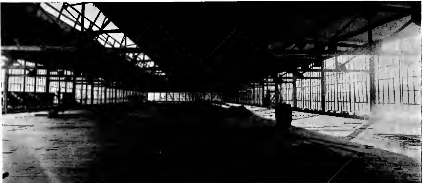
The upper floor of the new ship tool shed at Pusey and Jones' is utilized as a mould loft, one end being set aside for the draughting room.
